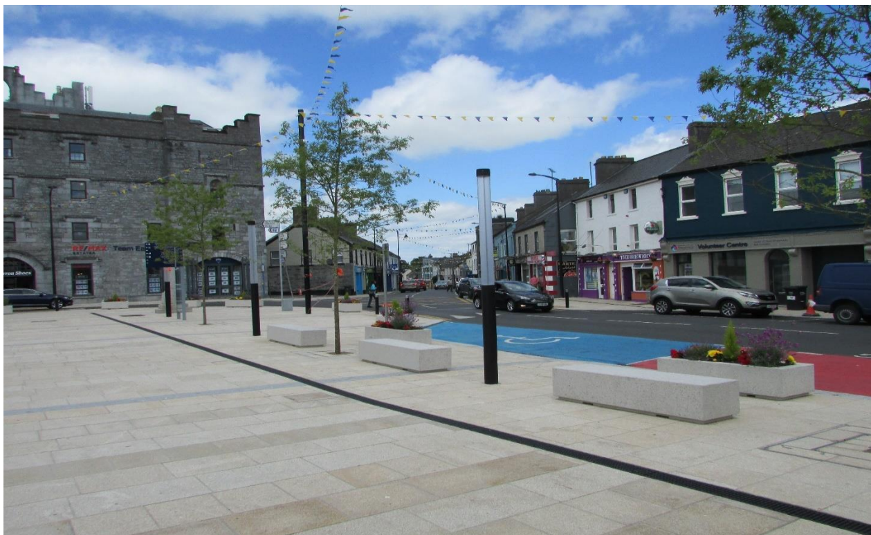
Public realm works in Roscommon Town
