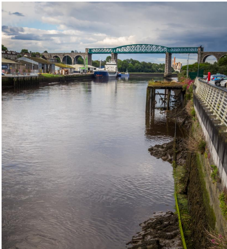
Boyne Viaduct, Drogheda
