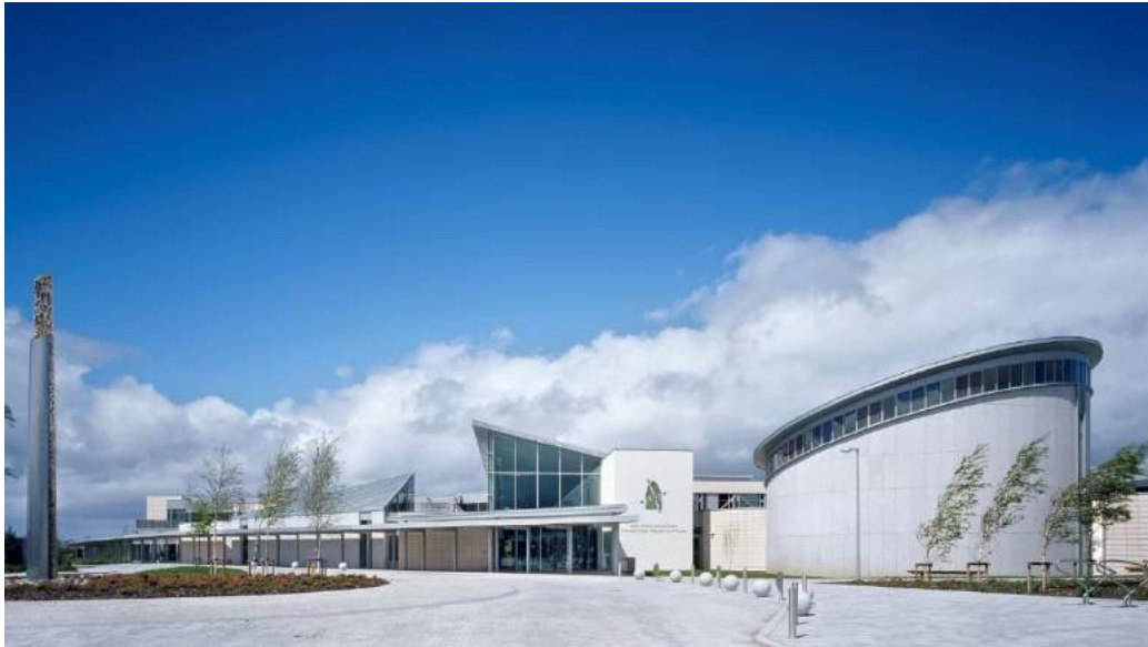
Tipperary County Council Civic Offices, Nenagh
